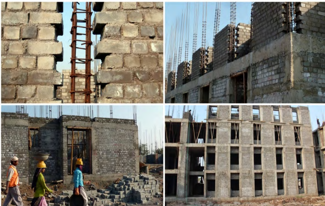
Fig. 9. Residential and hostel buildings under construction at IIT Gandhinagar, Palaj
