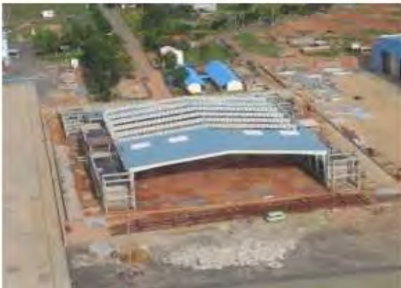
A VIEW OF STRUCTURE
