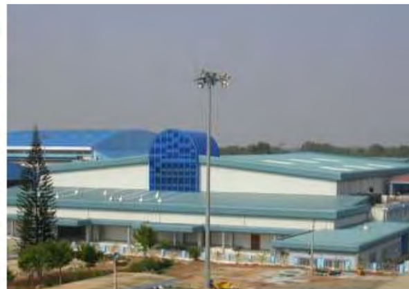
FRONT VIEW OF COMPLETED HANGAR
