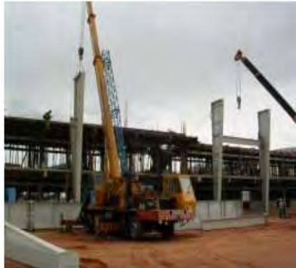
ERECTION OF RAFTERS
