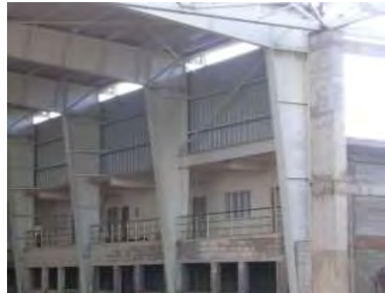
INTERFACE OF PEB STEEL AND RCC
