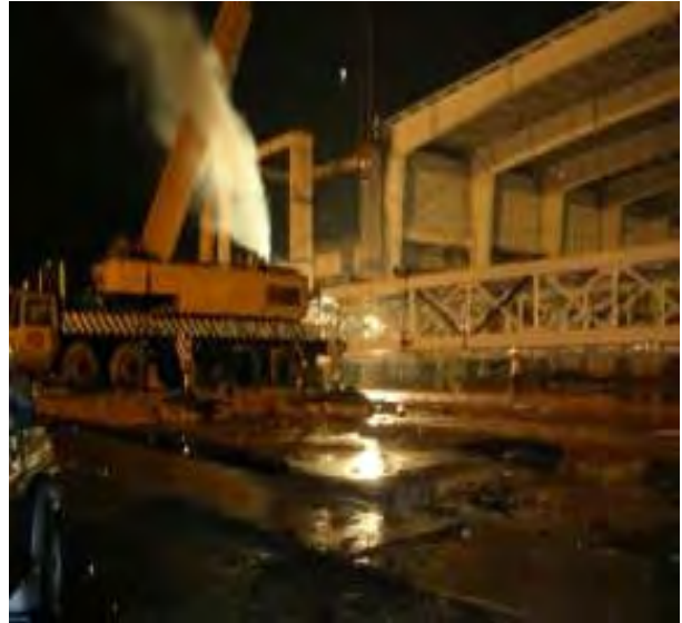
WIND GIRDER BEING ERECTED
