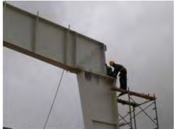
SETTING RAFTER OVER STANTION
