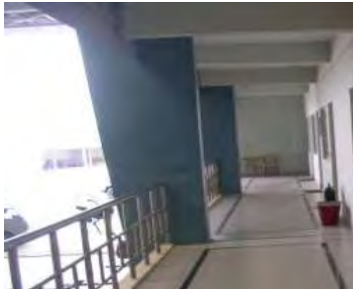
FIRST FLOOR CORRIDOR
