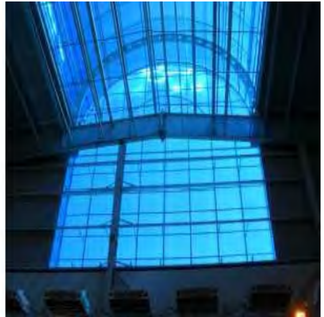
CLOSE UP OF POLY CARBONATE DOME
