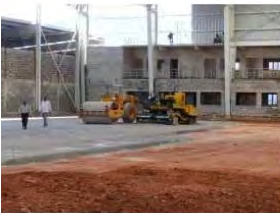
WMM IN HANGAR FLOOR
