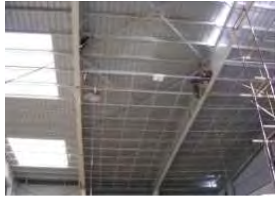
PANEL FIXED TO FLANGE OF RAFTER
