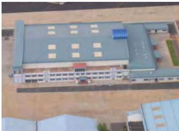
AERIAL VIEW OF COMPLETED HANGAR
