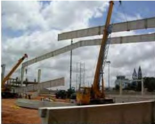
ERECTION OF END PORTALS
