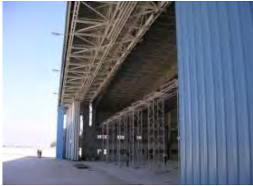
COMPLETED GATE STRUCTURE
