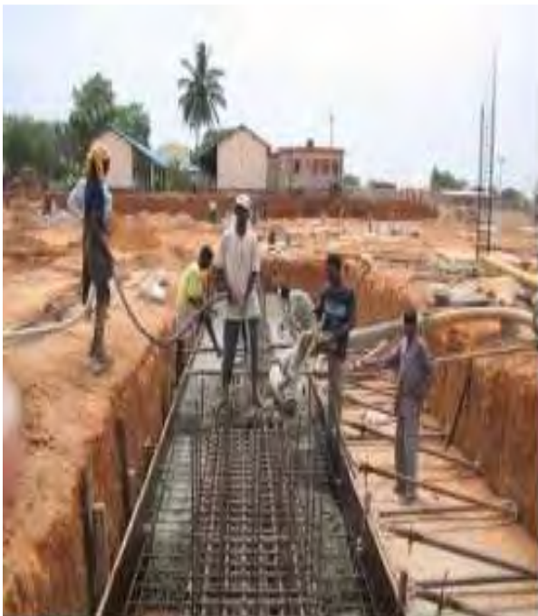
STRIP FOOTING BEING CASTED
